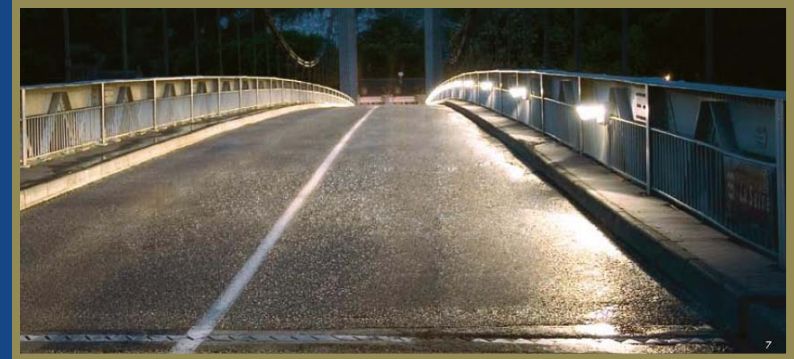
Low Profile Roadway Lighting Example
